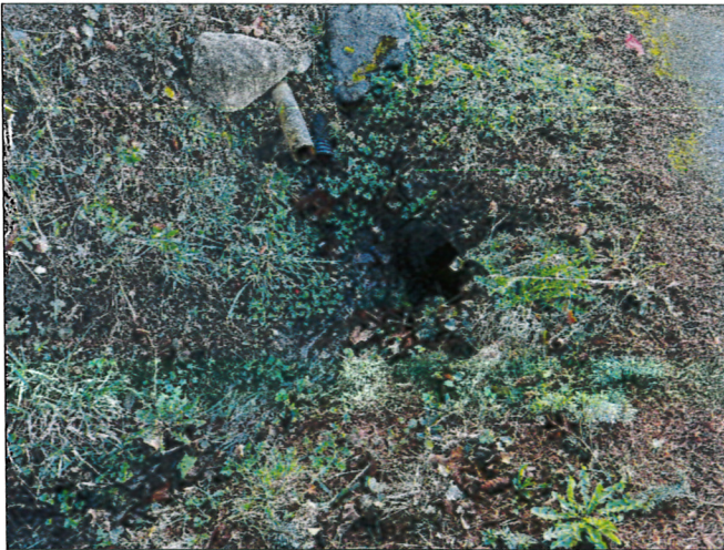
Photo 3: Stormwater drainage ditch culvert along SW corner of site.
