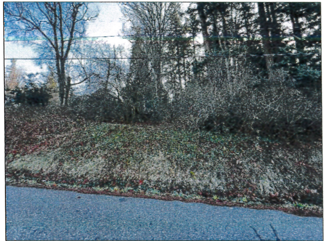
Photo 2: Road Cutbank along western frontage. Note grass covering and no exposed soils.
